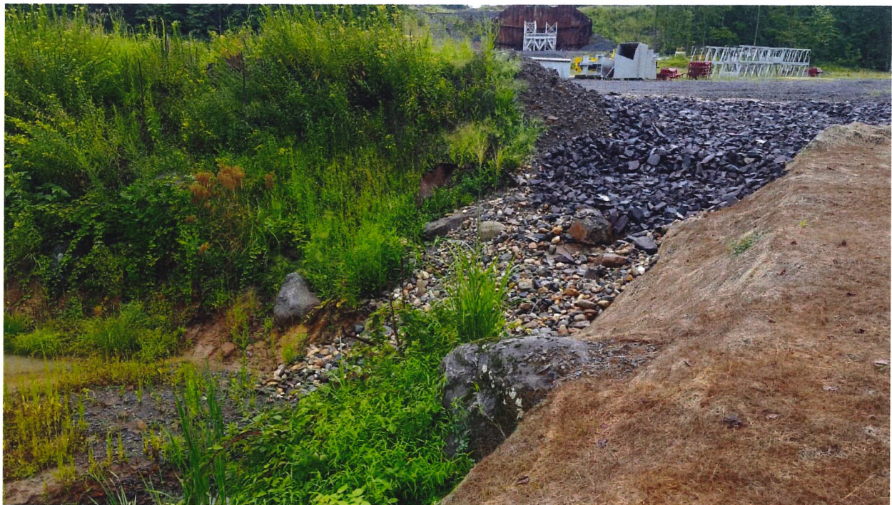
Photo #2: Standing on Southern berm facing Inlet Spillway #3
