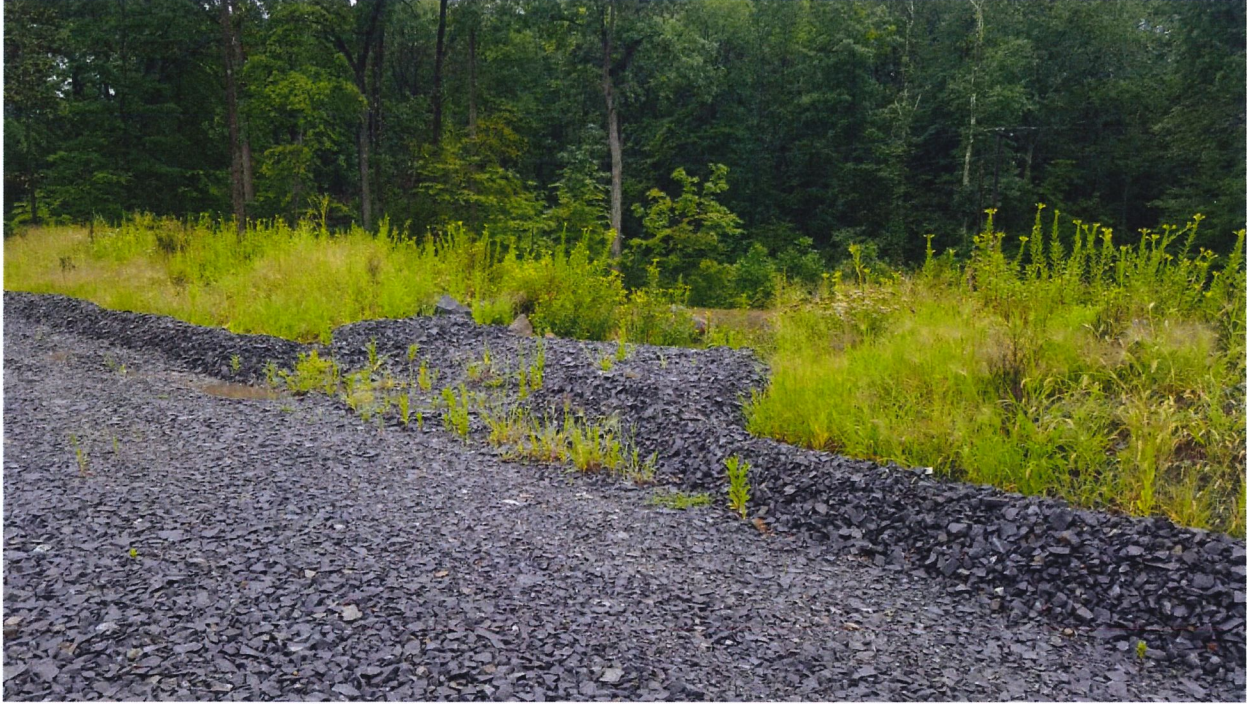
Photo #8: Looking at backside of Inlet Spillway #2
