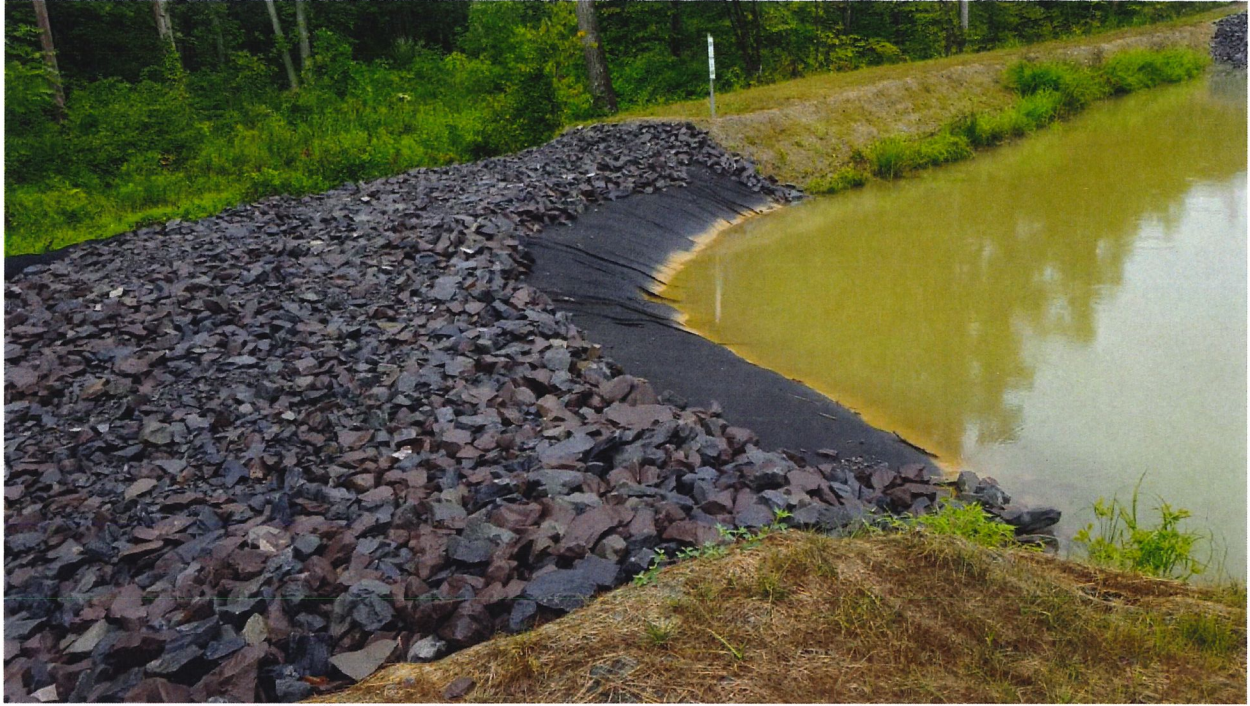
Photo #3: Standing on Southern berm facing Outlet Spillway
