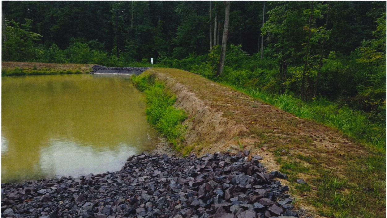
Photo #7: Standing on Inlet Spillway #1 looking at Western Berm
