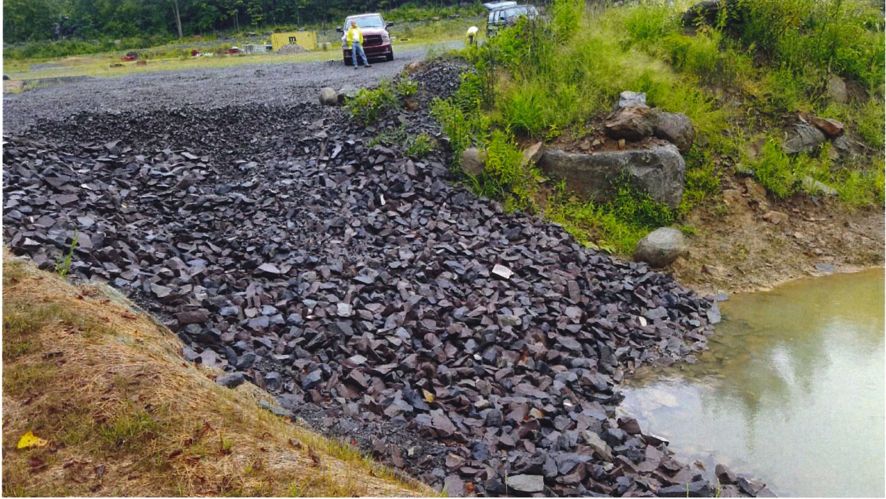
Photo #6: Standing on Western Berm facing Inlet Spillway #1
