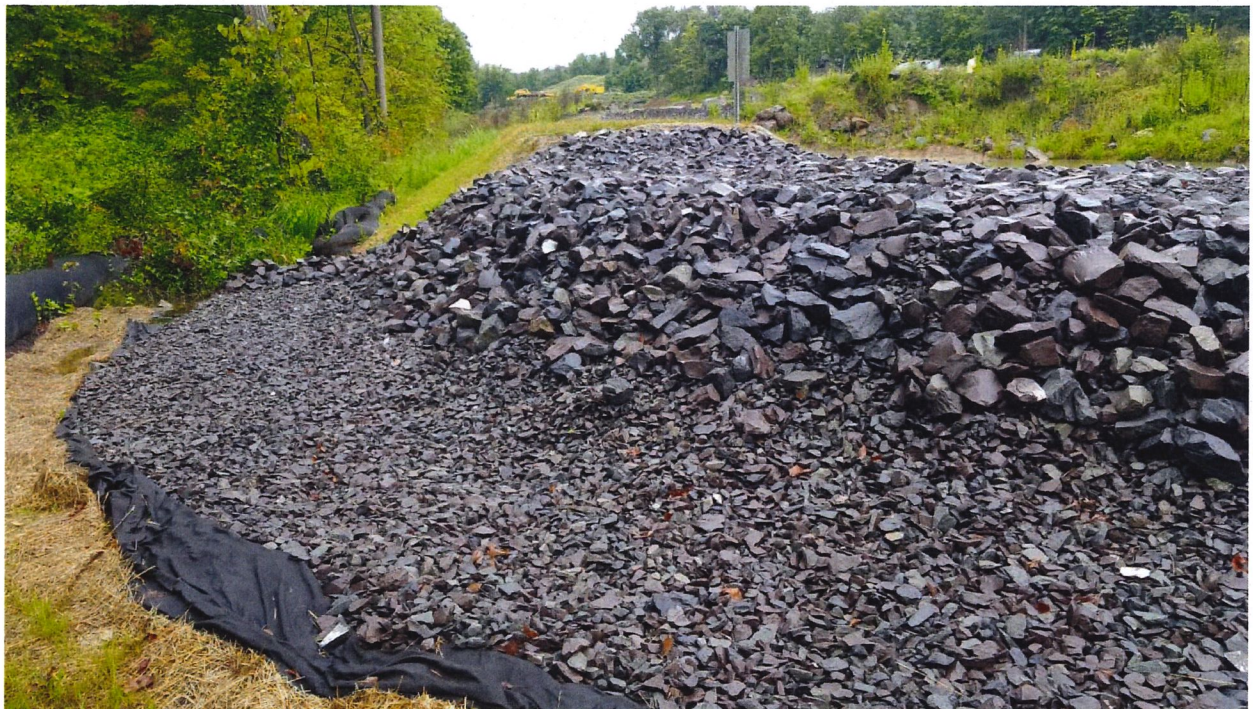
Photo #4: Back side of Outlet Spillway with Infiltration Trench
