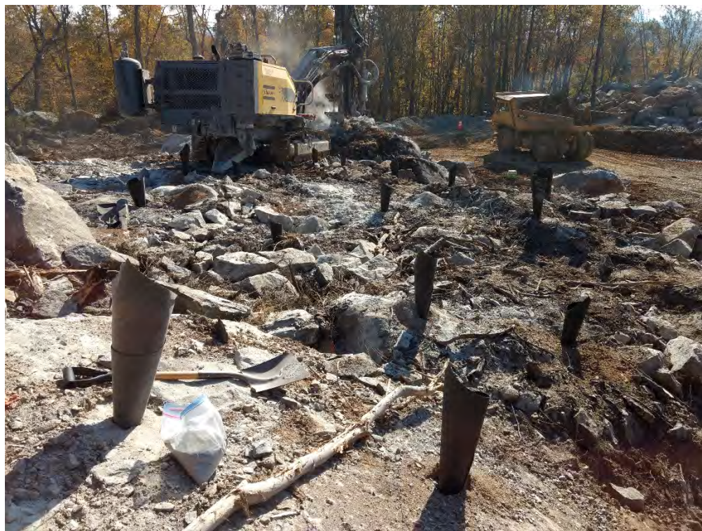
Photo 6 – S-7 and S-8 Drill Cuttings and Sample Locations
