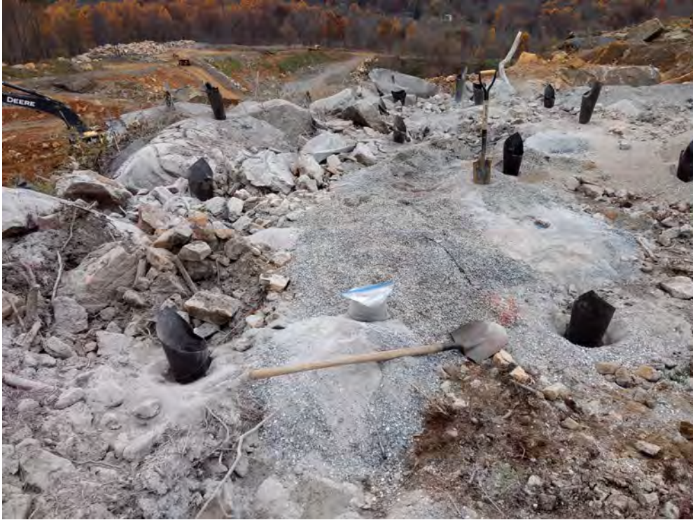
Photo 4 – S-9 and S-10 Drill Cuttings and Location
