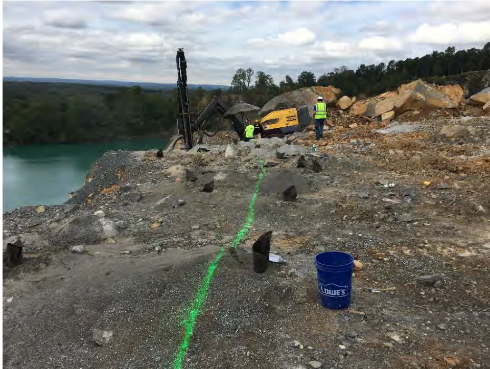
Photo 8 – S-11 and S-12 Drill Cuttings and Locations
