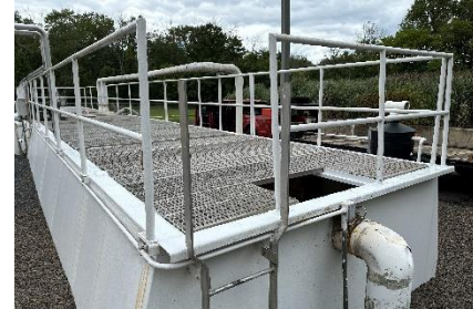
2023 Top of Treatment Tank Repair
