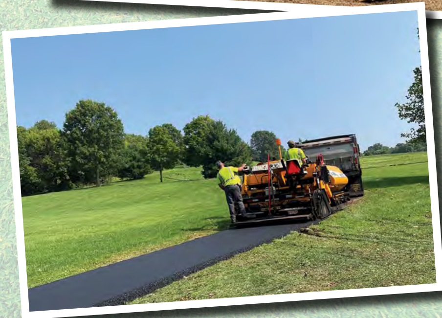
Photo at right: Walking trail in-house overlay at Iron Bridge Park, 1450 Branch Road
