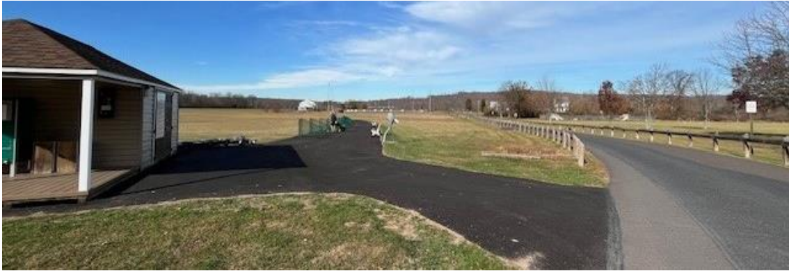
In 2024 the Golf Tee Area was Widened and Paved
