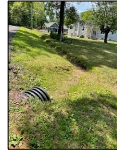
Storm Sewer ditch
